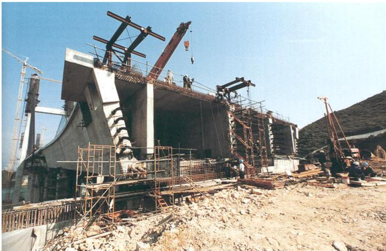
Lantau approach span launched into final position; probably the largest and stiffest incrementally launched
