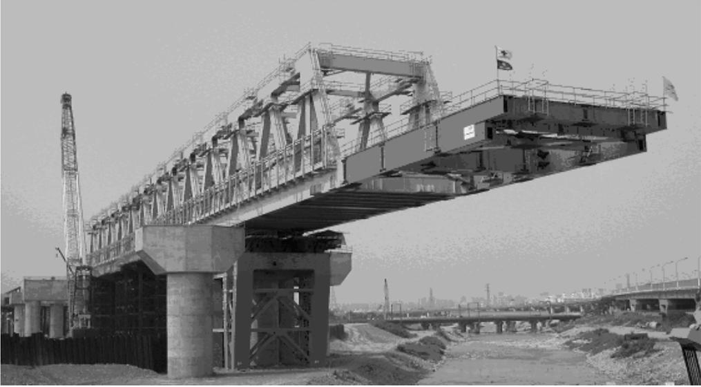
**Fig. 1:** Launching of a 3-span truss bridge.
