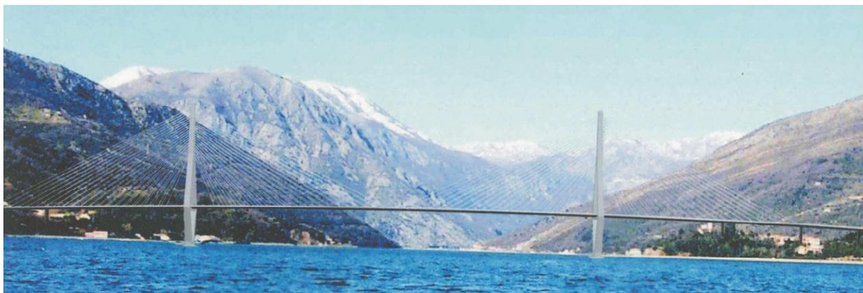
Fig.13 Verige Bridge, spans of 41+50+90+130+450+130+90m, Montenegro [4]
